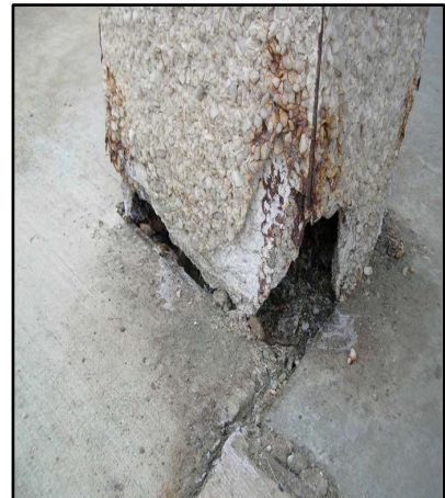
↑ Deteriorating aggregate stucco columns
