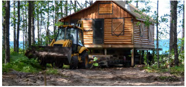
Relocating a cabin on Lake Superior, Luce County
